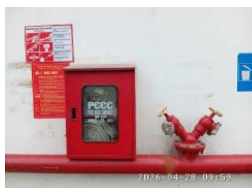
Fire hydrant and fire hose.jpg
